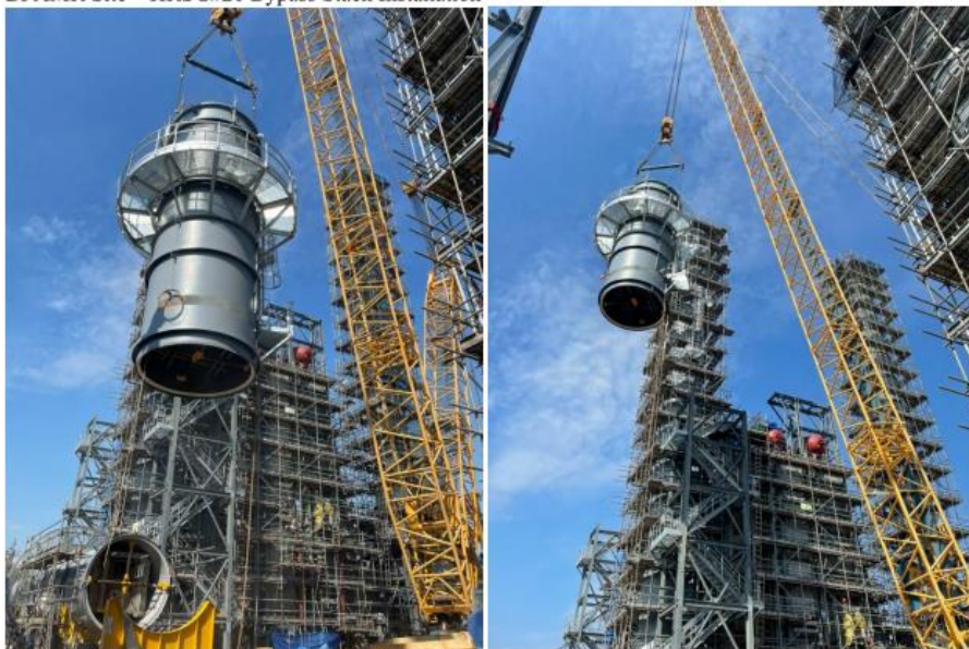
BPAMR Site – HRSG#21 Bypass Stack Installation
