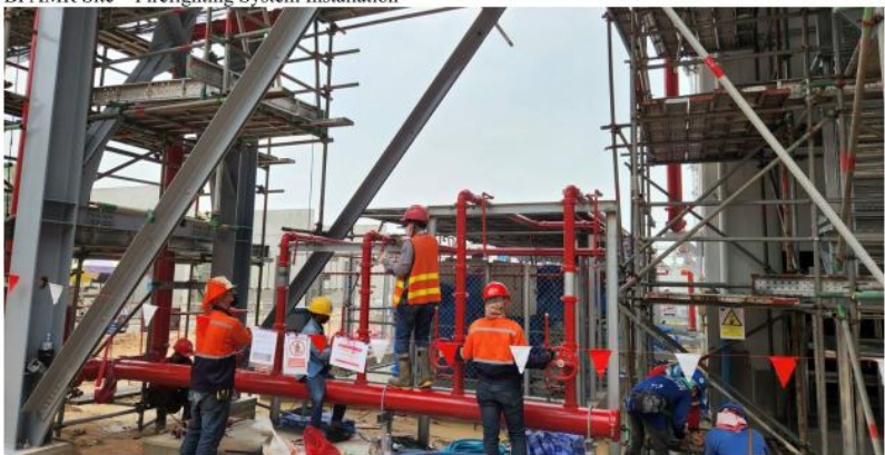
BPAMR Site – Firefighting System Installation
